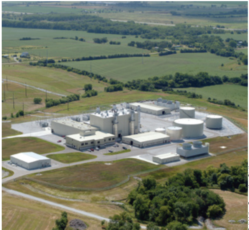
Salt Valley Generating Station
