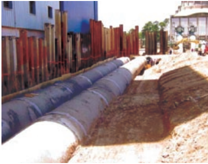
2. Circulating-water piping looking out to the cooling tower at the upper right of the left-hand photo; new concrete pipe at right attaches to a special spool piece to connect to the final section of FRP pipe near the condenser
