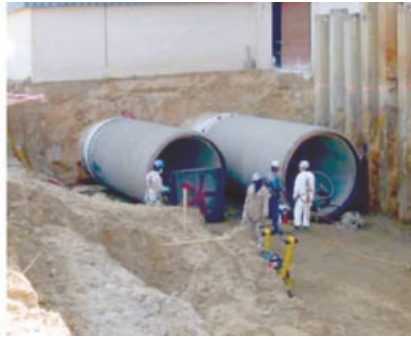
2. Circulating-water piping looking out to the cooling tower at the upper right of the left-hand photo; new concrete pipe at right attaches to a special spool piece to connect to the final section of FRP pipe near the condenser
